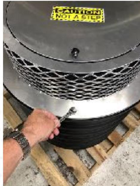
Prior to installation remove the Top-Hat-Filter from the Pre-Fab Petro-Barrier by removing the 2 Hex Head brackets that hold the THF in place.
